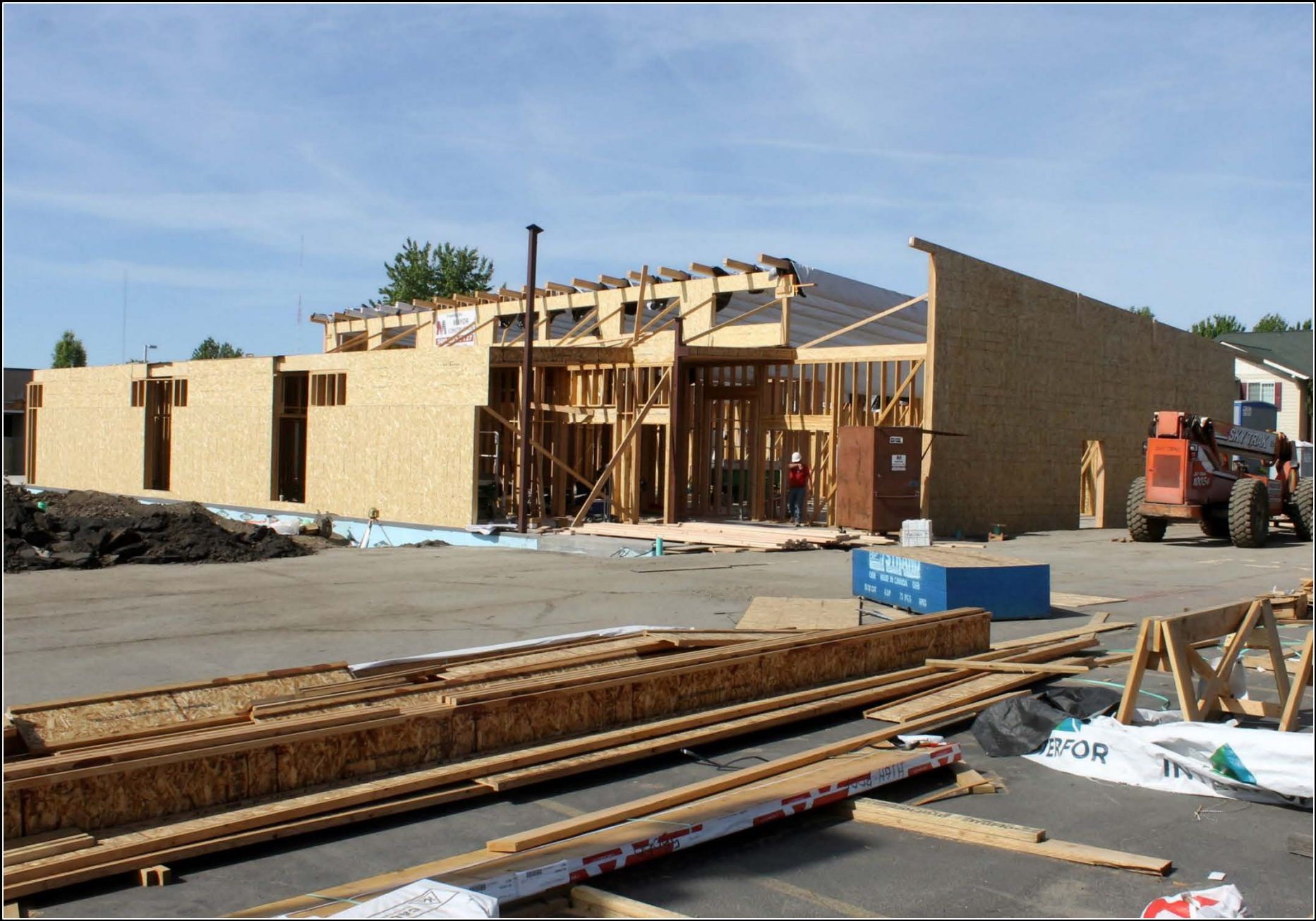
Front view (future building entrance): East wall, left; north wall, right
