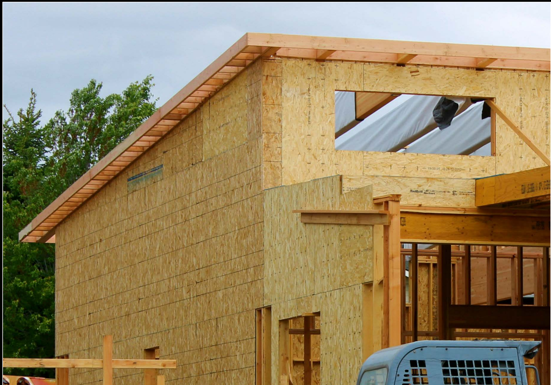
Soffit work begins
