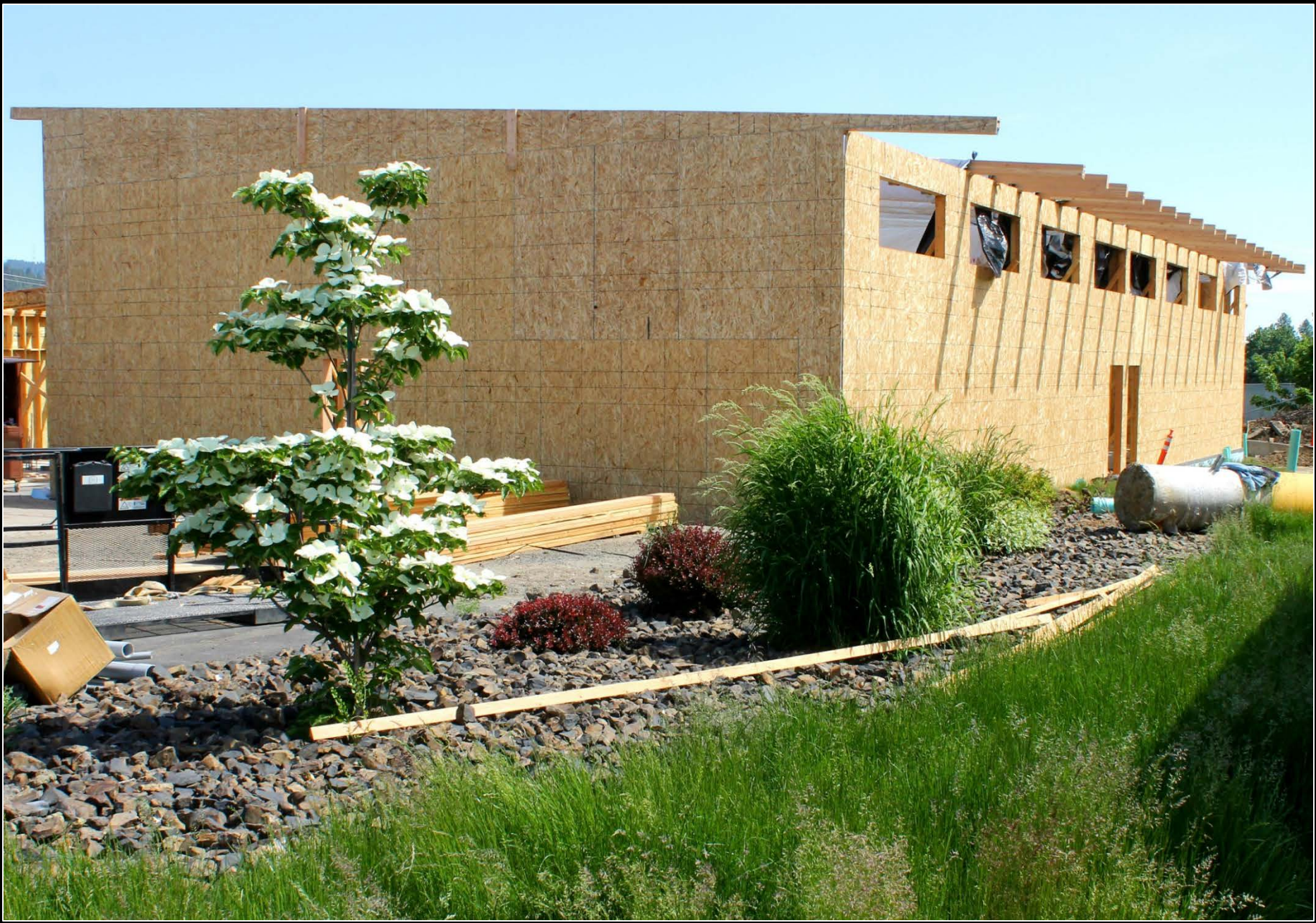
Rear view: West wall, left; south wall, right
