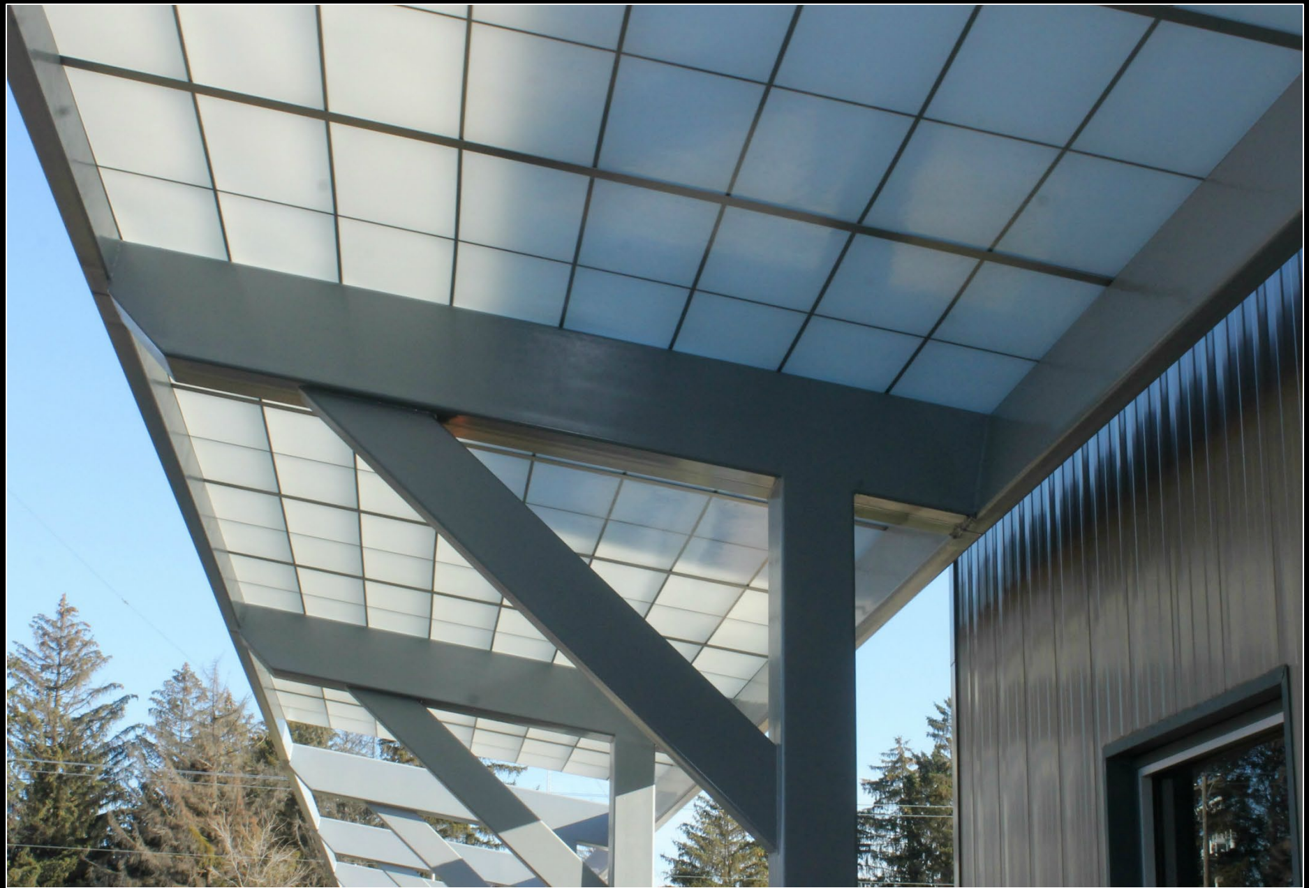
Covered walkway connects conference center to NEWESD 101 offices
